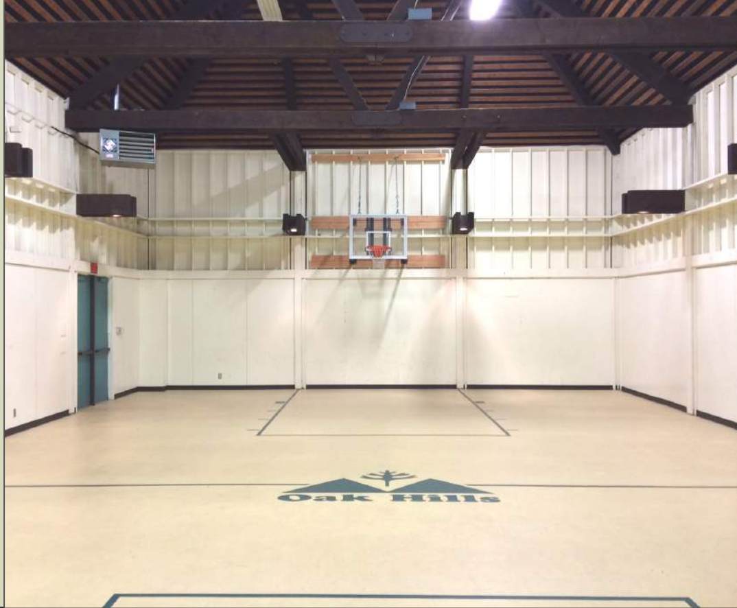
EXISTING CONDITIONS - GYMNASIUM
